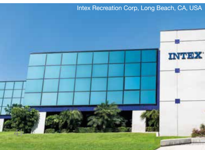
Intex Manufacturing and Distribution Complex, Xiamen, China
